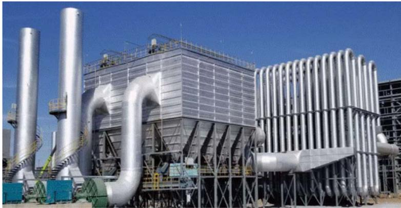
The room-cleaning bag filter has the characteristics of large air volume, compact structure, small floor space, less steel consumption, low energy consumption and convenient operation and maintenance. Dust emission concentration  $\leq 30\text{mg}/\text{m}^3$
